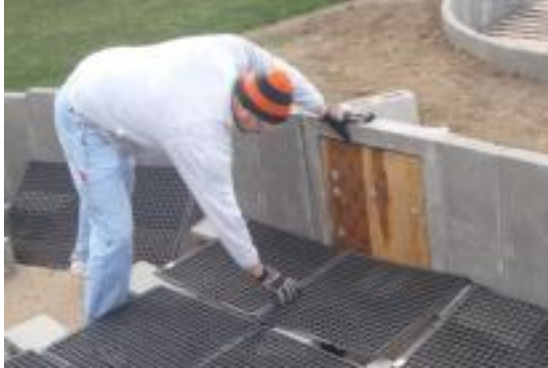
Matt Robert places poultry flooring in biofilter
